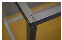
Figure 7: The rectangular frame is constructed from 1/2 in. square aluminum stock. A single 10-32 flathead screw secures the three interlocking pieces that form each corner.
